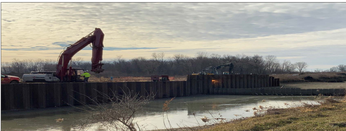
PIP-II Fermilab construction coordinator observing the sheet pile wall installation for the site work phase. Credit: Steve Dixon
