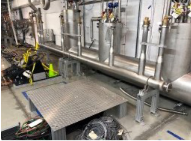
Disassembly of PIP2IT and installation of cryogenic transfer line for the 650 MHz Test Stand.
