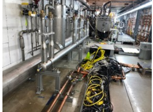
Disassembly of PIP2IT and installation of cryogenic transfer line for the 650 MHz Test Stand.
