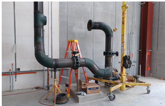
ICW piping installation underway
