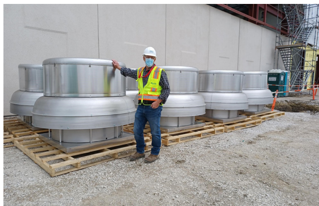
ODH fans staged for installation
