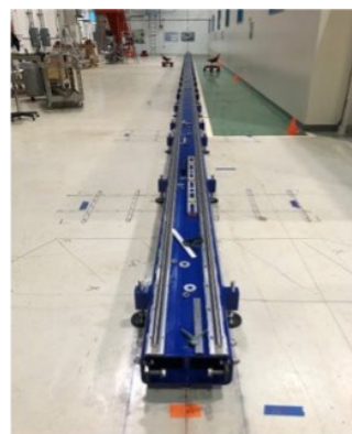
MP9 cleanroom rails installed, alignment underway
