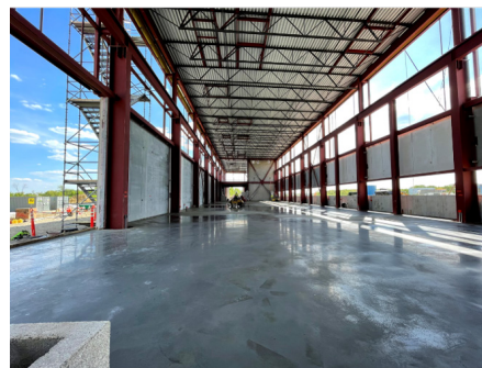
Warm Compressor Station floor slab, 14 May 21
